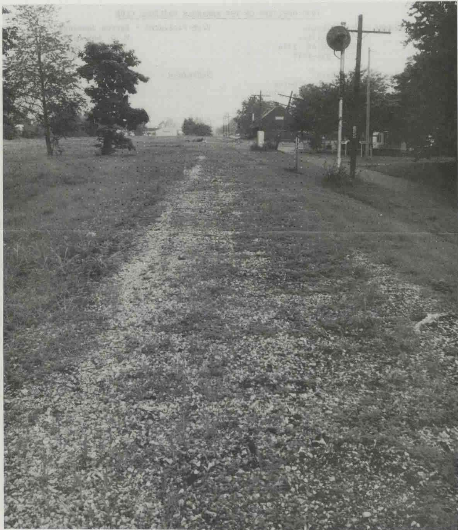
Looking east along the old Rock Island's abandoned "Sunbelt" main line in North Little Rock. Rock Island's Argenta depot is to the right. The photo was taken on a cool, drizzly day in the spring of 1989 by Ken Ziegenbein.
