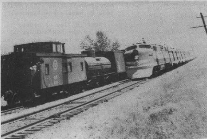
TOP- SLSW #819 on her maiden test voyage April 17, 1986 in Pine Bluff after being rebuilt in the same Pine Bluff shops in which she was originally constructed in 1942. BOTTOM - One of Mr. Rudolph Diesel's machines heading a MOP passenger train, location unknown, in the late 40s or early 50s. (Top photo - Ken Ziegenbein; Bottom photo from the collection of William Church).
