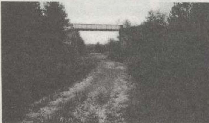
B&N bridge over the now-scraped Rock Island tracks in Bauxite. (September, 1985 photo)
