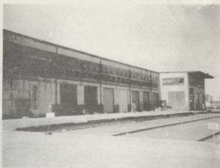
SSW Steam engine #819 is being restored in this building. On this date, the locomotive was 81% complete.
