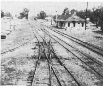
This switch is in the Kansas City Southern yards at Ashdown, about a block north of the KCS depot. One switch stand throws all four sets of points, so regardless which way a train enters, the switch won't be hurt. The problem is knowing which way to come out. As the switch stand has no light or target, it is a puzzle for the brakeman to line the switch for the right track. Such switches are fairly common in congested big city terminals but are rare in southwest Arkansas.
