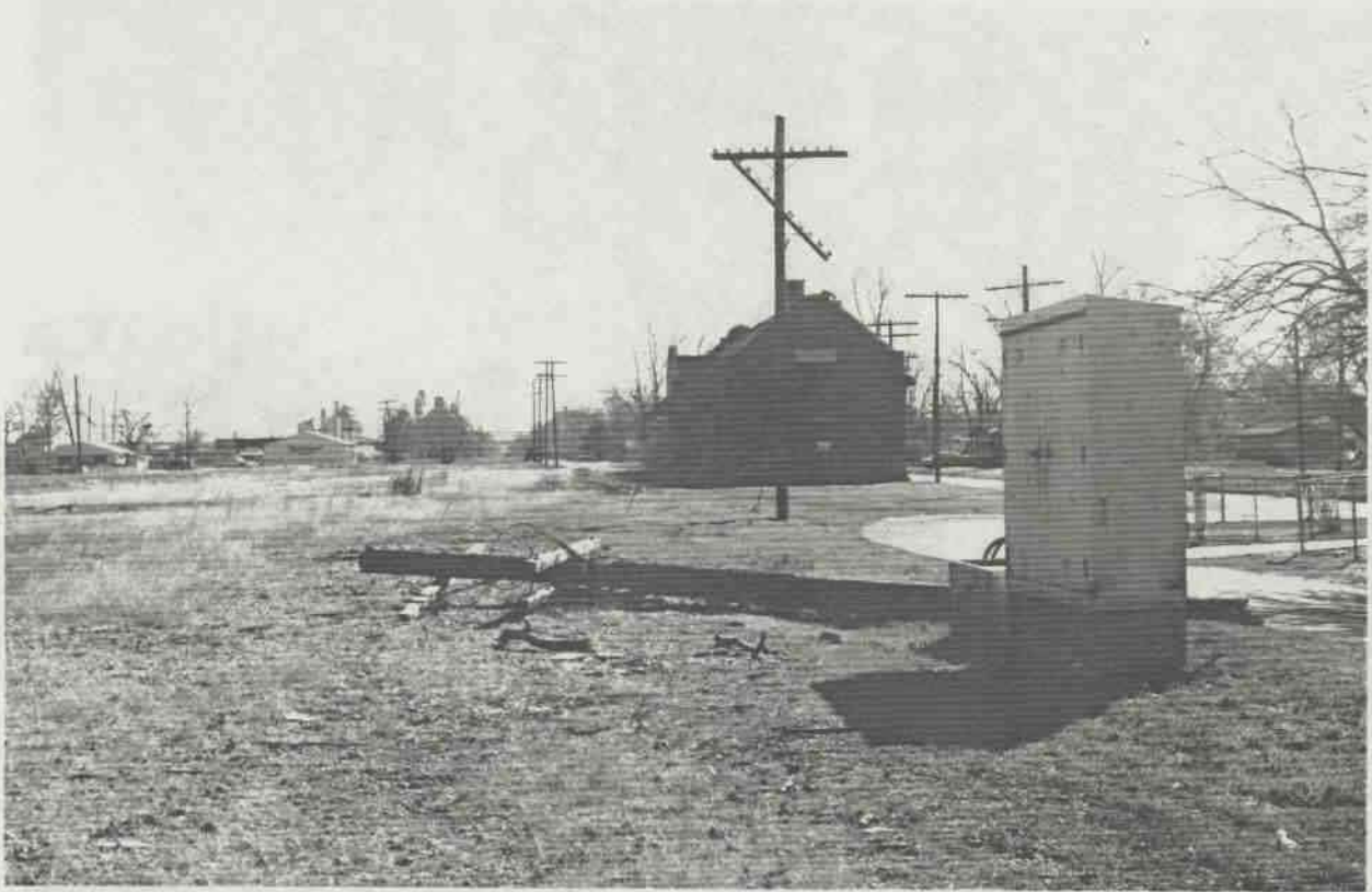
In the foreground the signal control box is empty and rusty, the fallen skeleton of a telephone-telegraph pole lies where it fell. The deteriorating brick depot with its red tile roof is home for ghost railroaders. The few remaining poles, one with a sagging crossarm, resemble an ancient, snaggle-tooth grin. The North Little Rock (Argenta) area of THE ROCK is a sad scene, indeed. (March 1991 by Gene Hull)
