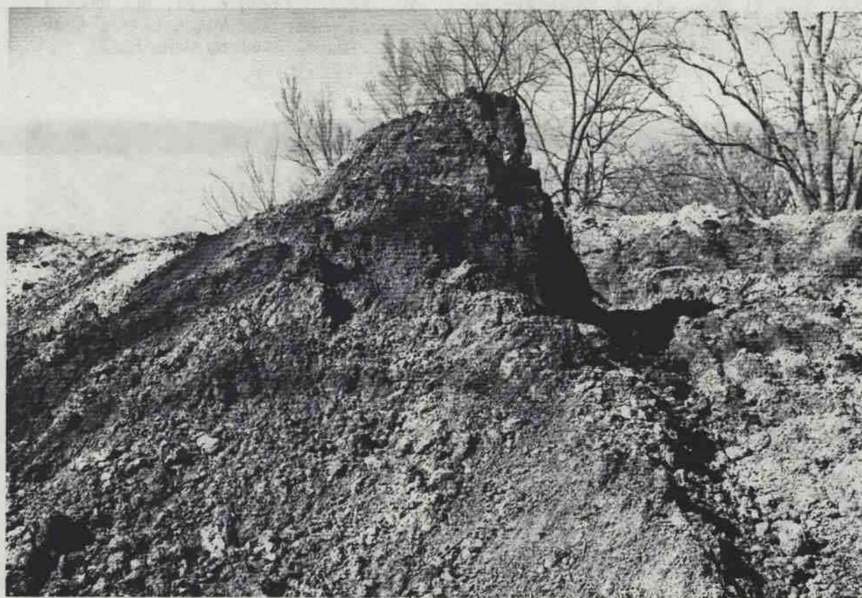
TOP - This heavy earth-moving equipment is quickly removing all vestiges of the Rock Island embankment in North Little Rock north of the Arkansas River bridge. (Gene Hull photo, March 1991). ABOVE - Just south of East 2nd Street in North Little Rock the Rock Island track embankment was about nine feet high. This material was sold to Edward Epperson, a professional house mover, and Harvey Townsend. As heavy, earth moving equipment began loading and hauling the material, this hummock revealed the upper two feet was composed of cinders from early coal-burning locomotives. (Gene Hull photo, March 1991)
