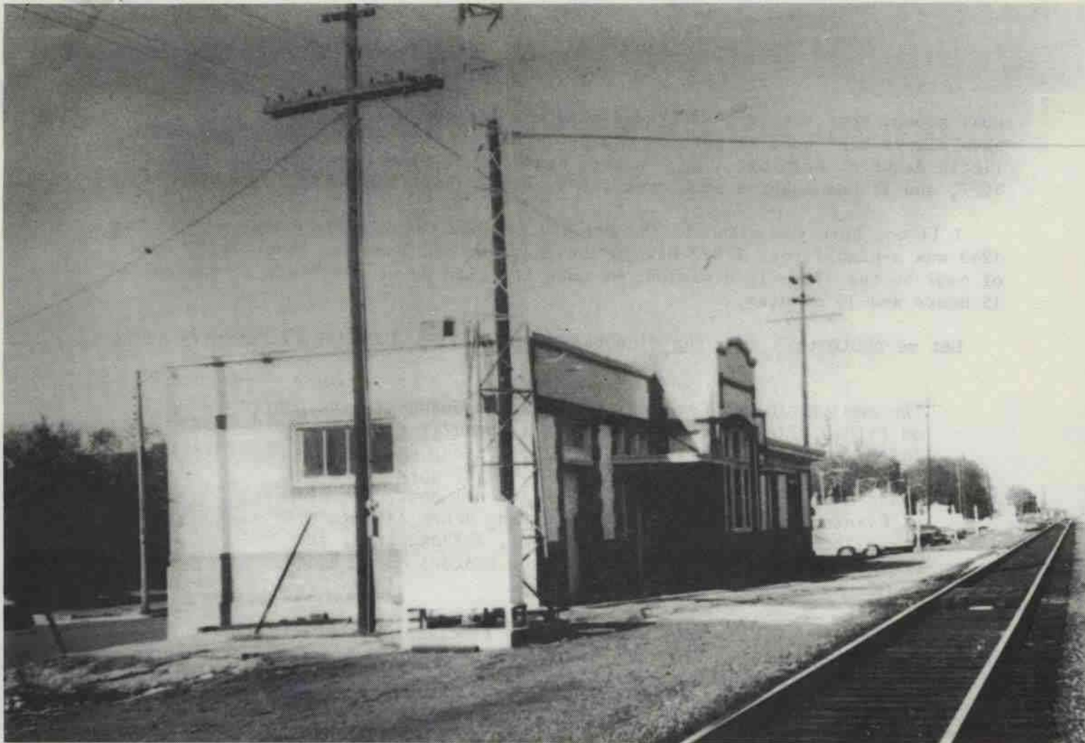
UNION PACIFIC (Missouri Pacific) Corning, Arkansas depot, taken in the late 1960s. It was opened in January, 1927 and is to be given to the city of Corning. (E.A. Hille)
