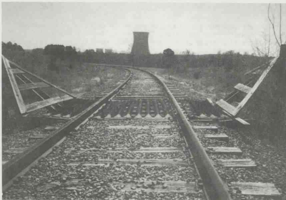
After seeing Bill Bailey's story on the KCS's last cattleguards in the April RAILROADER, Steve Couch of Russellville spotted this cattleguard on the Union Pacific's Arkansas Power & Light spur track to the Arkansas Nuclear One power plant just south of London, Arkansas. The plant can be seen in the top center. (Steve Couch photo, April 1988)
