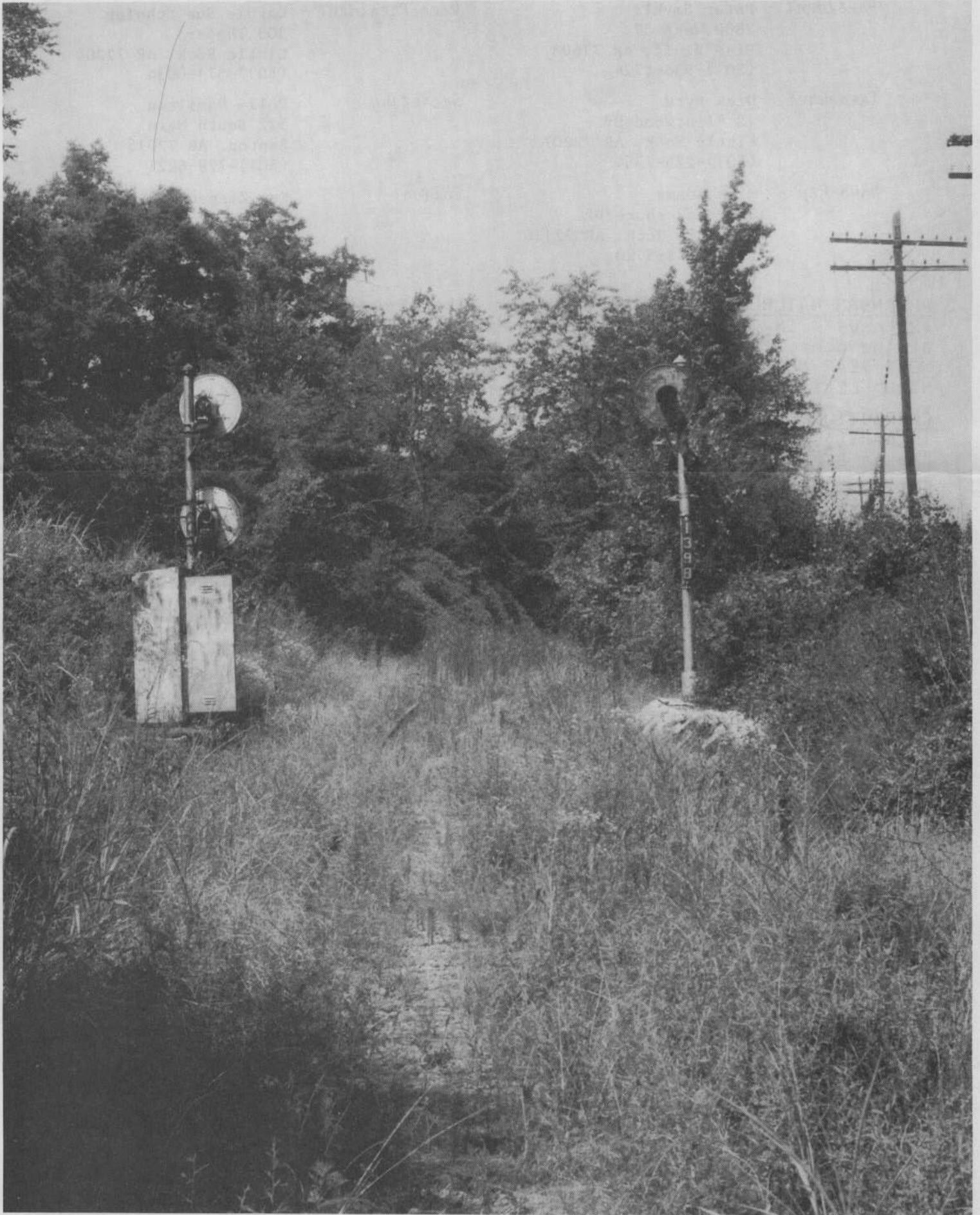
PROTECTING GHOST TRAINS, these signals along the abandoned Rock Island just west of Union Station in Little Rock keep the vigil...just in case. Photo taken in August of 1985 by your editor.
