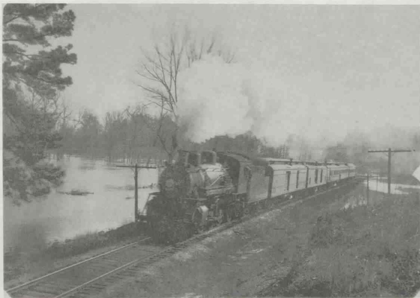
TOP - A Rock Island passenger extra with 7 cars, pulling out of the Rock Island Yard at Camden, Arkansas in 1938. This was a football special carrying the Camden Panthers to Hot Springs to play the Trojans. The RI had trackage rights on the Cotton Belt from North Camden to Kent, two miles, then switched back to the Rock Island. This two-mile area was covered largely by bridges and trestle work across the Quachita River bottoms and was subject to overflow about every year. Notice the SSW coal chute on the left. BOTTOM - A Missouri Pacific passenger train three miles north of Camden bound for Gurdon about 1935. (P.B. Wooldridge photos)
