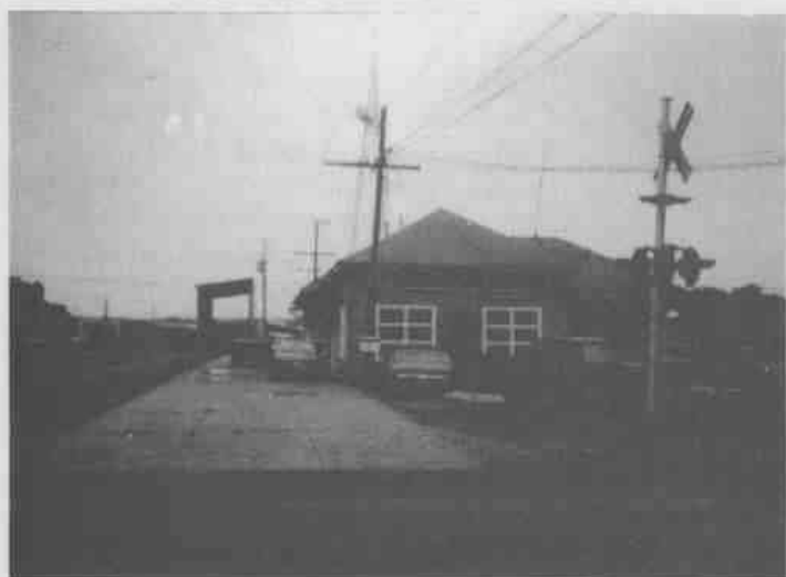
D&E depot in DeQueen, Arkansas looking west.
