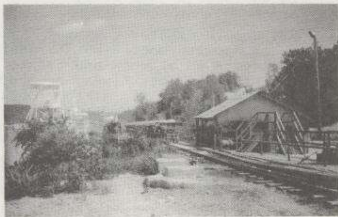
View of the kilns after a load of crushed stone arrived.
