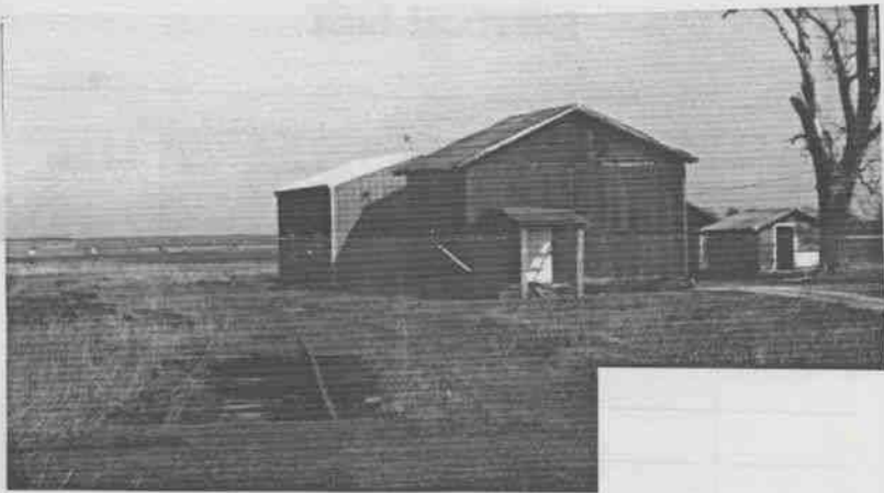
← The old roundhouse at the south end of the yard. Note the old engine inspection pit in the foreground.
