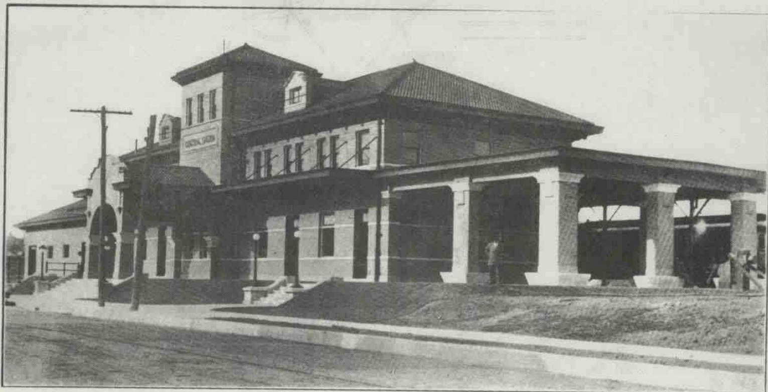
Central Station shortly after its 1911 opening. This impressive structure was owned by the L&A, but used also by the Cotton Belt. The trolley line on Marshall Street was conveniently accessible to L&A/Cotton Belt patrons. (Author's collection)
