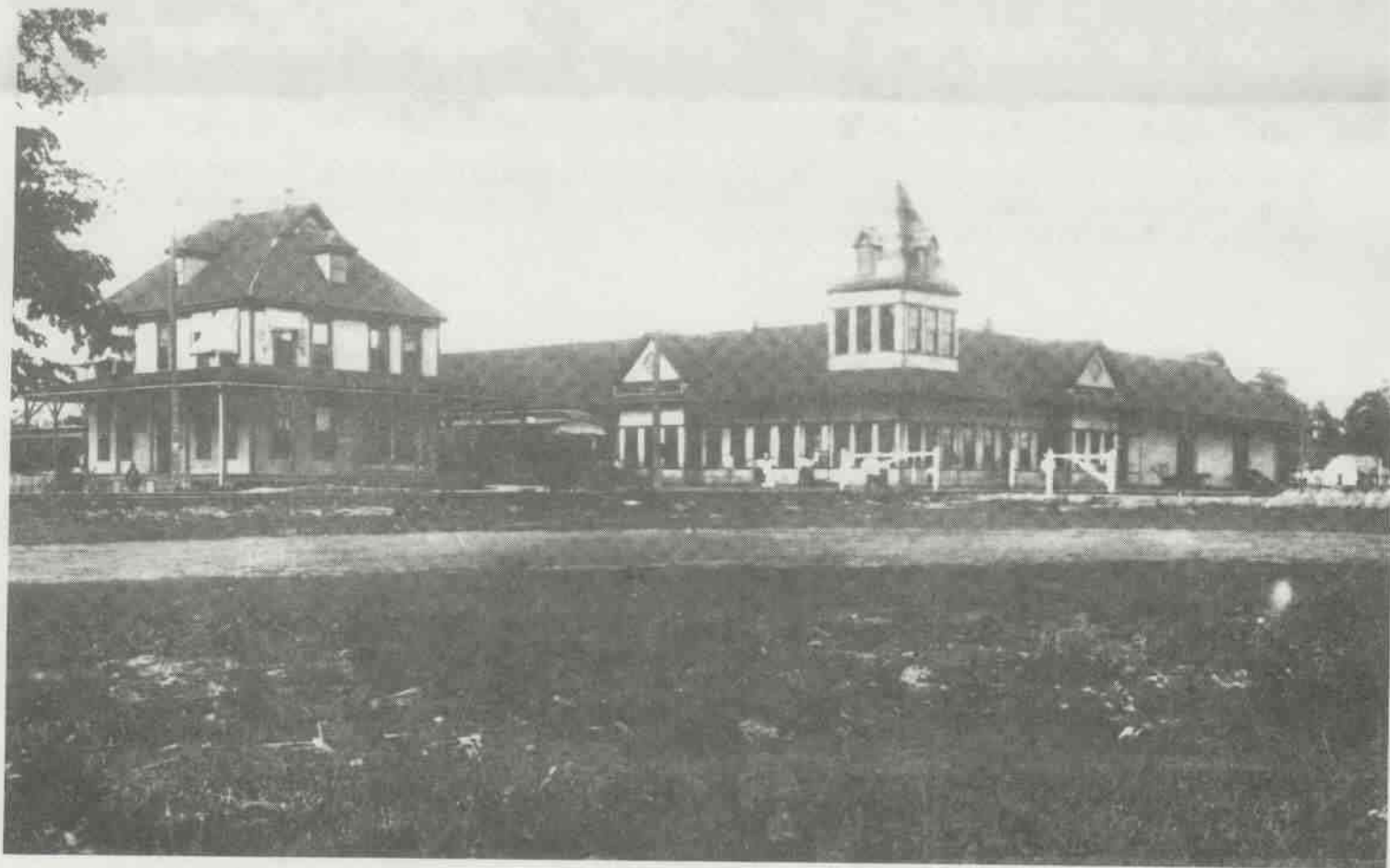
Stamps, Arkansas union station in 1904. Headquarters building of the L & A is at the left. The passenger train is northbound on the L & A, just ahead of the Cotton Belt crossing, and appears to have William Buchanan's private car, "The Bodcaw", at the rear. (Author's collection)
