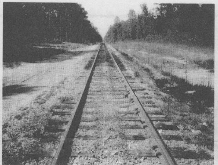
Although difficult to see in this photo, long stretches of the Ashley, Drew & Northern between Crossett and Monticello have a roller-coaster look. Not much grading was done when they wer laid.
