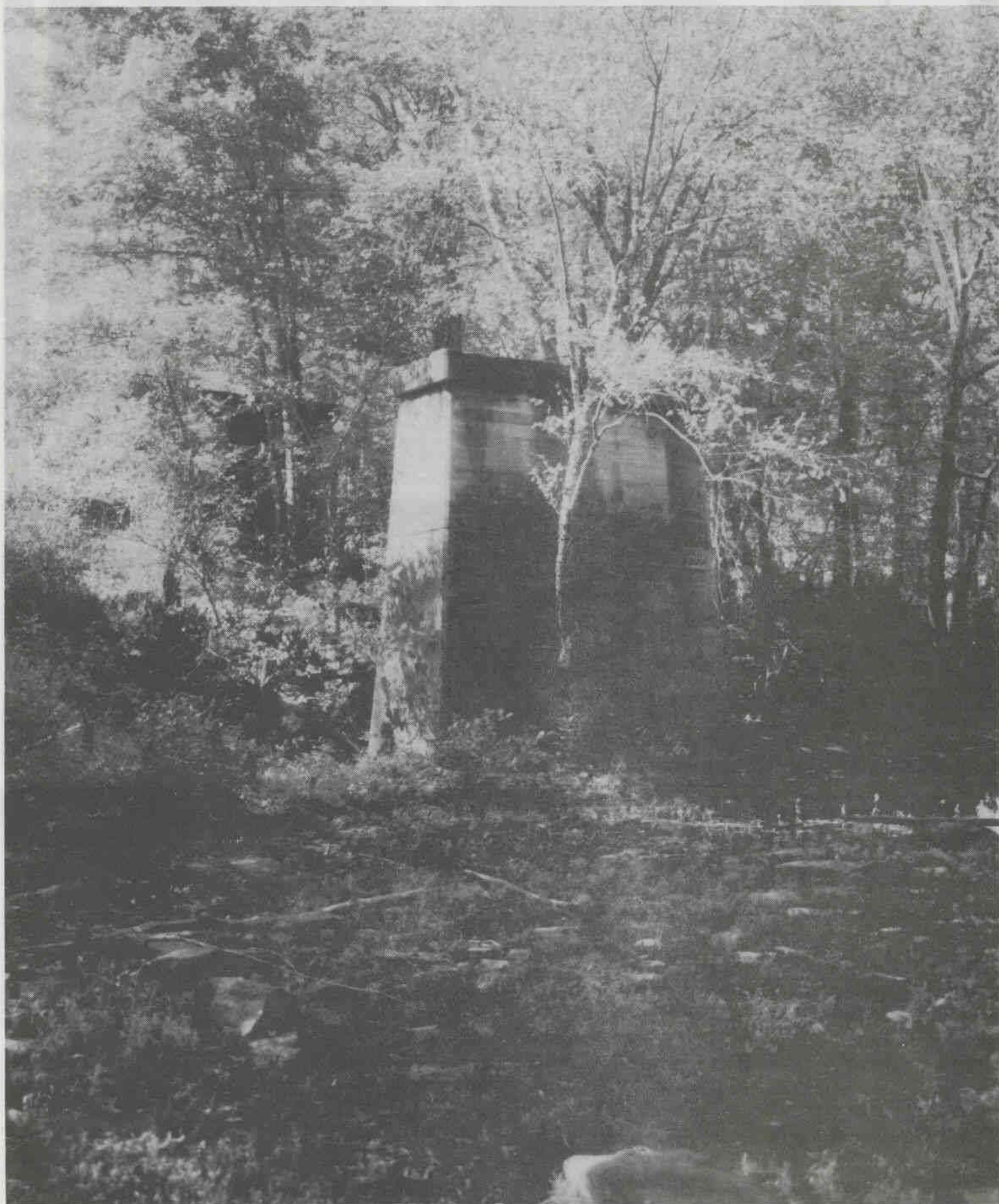
OLD M&NA bridge pier over Big Creek between Pangburn and Letona, Arkansas taken on October 10, 1991 by Doug Duncan. There remain many traces of this famous line in Arkansas, even though rails were taken up in the 1940's. (Doug Duncan photo)
