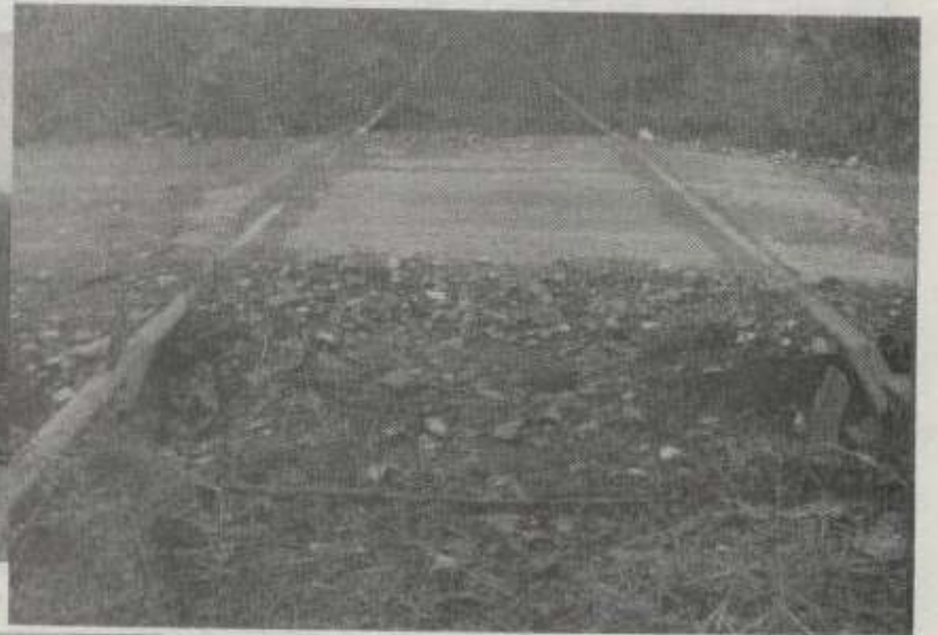
ABOVE LEFT - While one crew loosens the rail, another picks the rail up with this magnet and stacks the pieces neatly along the side. ABOVE - Rails are broken and bent at road crossings before the dozers get there, as at this crossing east of Hartford. LEFT AND BELOW LEFT - A 2-man crew moves along at about 8 miles a day undoing a railroad that's been there for 100 years. The dark storm clouds were befitting to the occasion. (Photos by Ken Ziegenbein, November 19, 1985)
