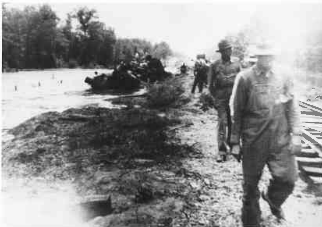
A KCS wreck of a caboose hop caused by a washout at Bridge A 453 (Flat Creek) just south of Winthrop, Arkansas circa 1943. Brakeman Frank Huckabee of Texarkana was killed in this wreck (he drowned). (Philip L. Moseley photo)
