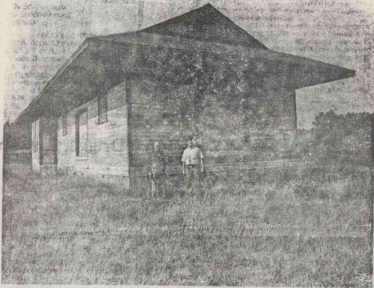
To restore depot...Coles, Jones look over old railroad depot at Coles' ranch near Glenwood
