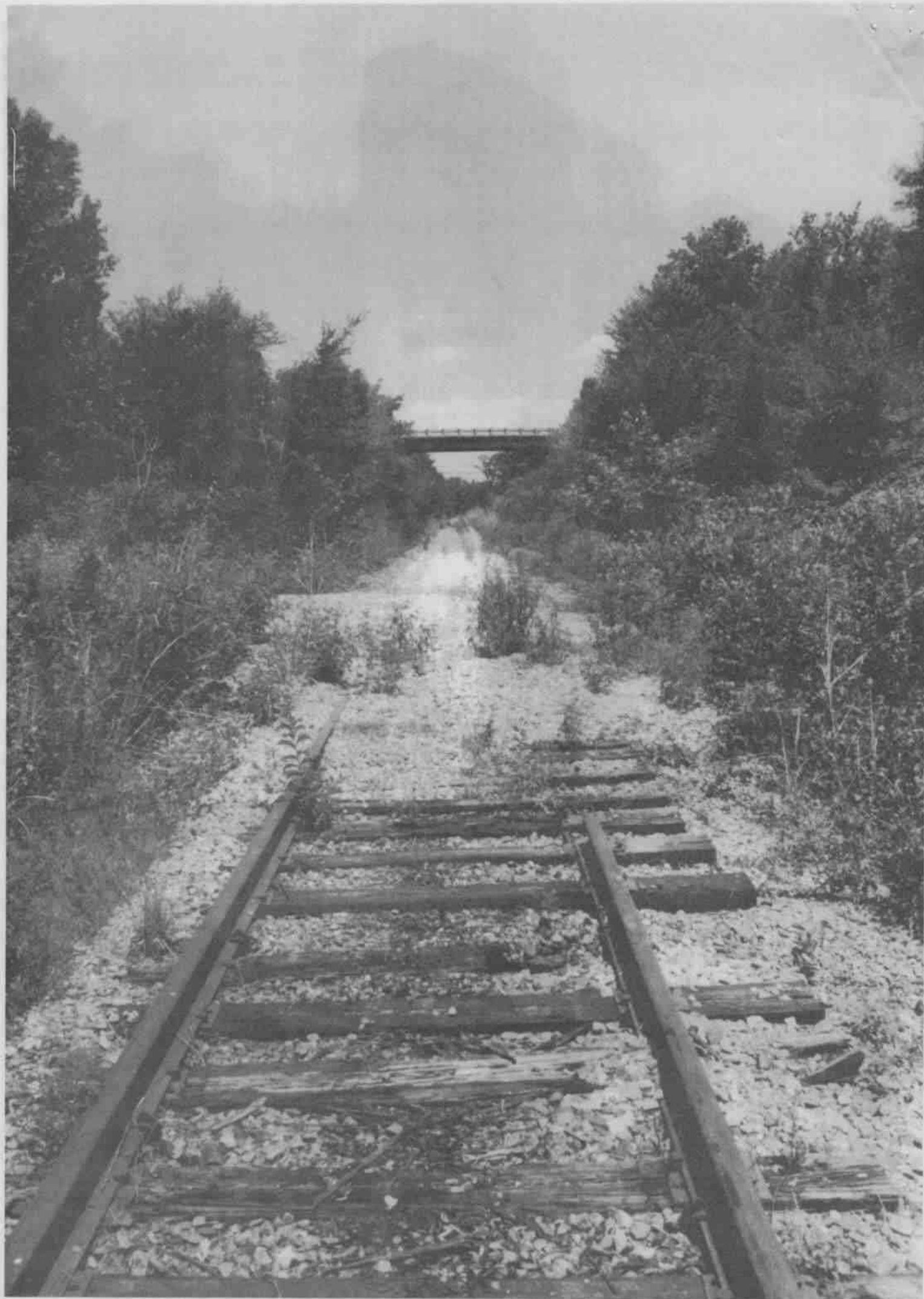
END OF THE LINE - Gone, except for the memories, is the Rock Island Sunbelt Line west of Danville, Arkansas. The line from Danville to Howe, Oklahoma was taken up earlier in 1986 by L. B. Foster with many of the rails now stacked nearby this location. The overpass is Arkansas Highway 27 about a mile west of Danville. (July 16, 1986 photo by Ken Ziegenbein)
