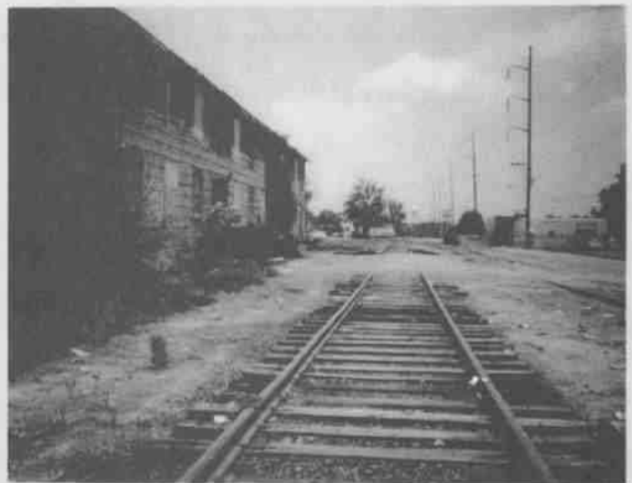
The original tracks of the Missouri & North Arkansas still exist through south Searcy. The DK&S uses these occasionally. The tracks end about 1/4 mile behind the photo (to the west).
