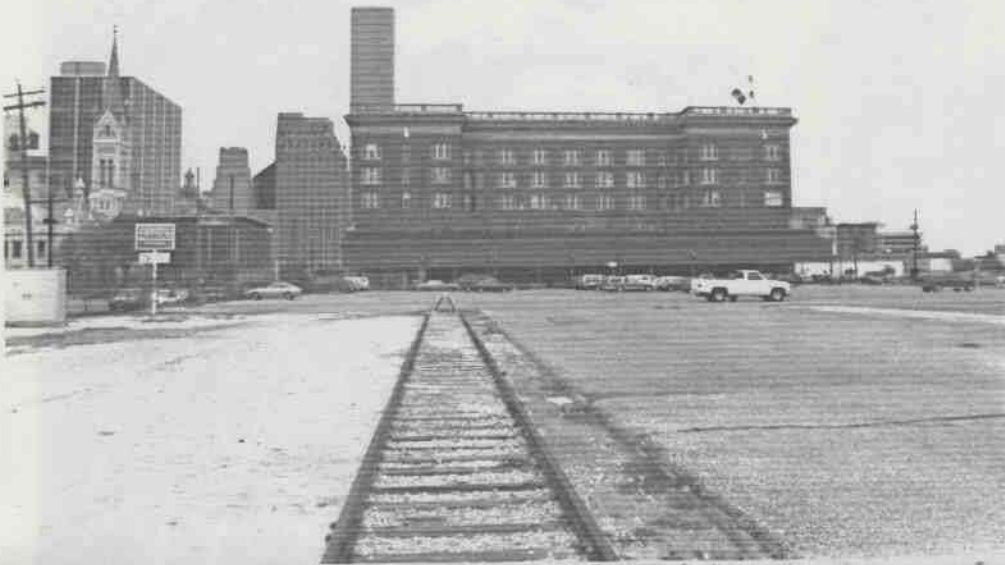
Only a single track remains of what was once many more. Santa Fe, Missouri Pacific and others once used this station...even Amtrak in the early 1970's. Trains would back into the station.
