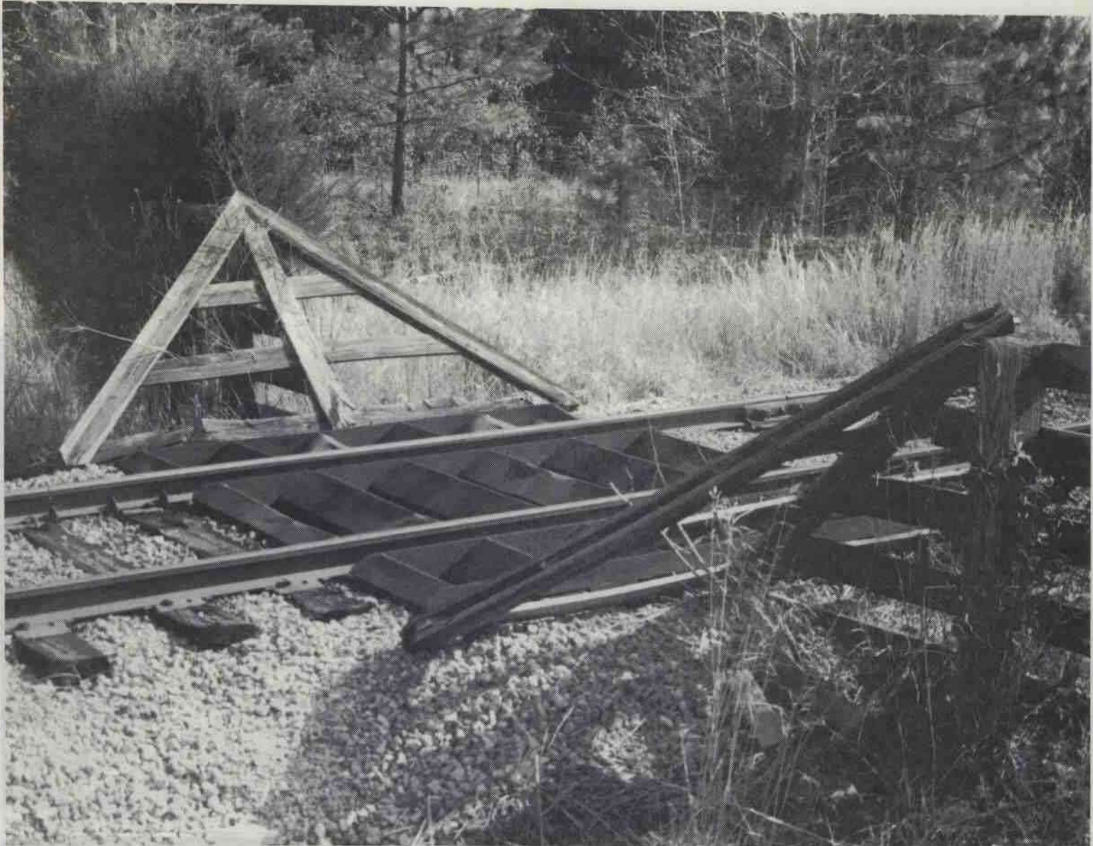
LOUISIANA & ARKANSAS RR cattle guard still maintained by the railroad on the Texas sub-division between Newsome and Pickton, Texas on service track into the old Tidewater Refinery Works. (Bill B. Bailey photo - December 29, 1987)
