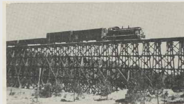
Picturesque Trestle on AW to Be Abandoned
